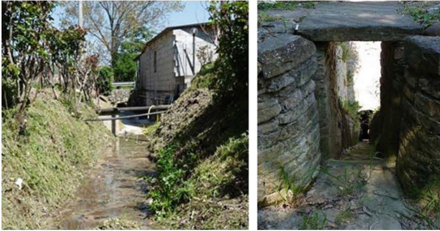
Fig. 6 Soil diversion channel photos. On the right , the last stretch of the channel, just upstream of the mill
