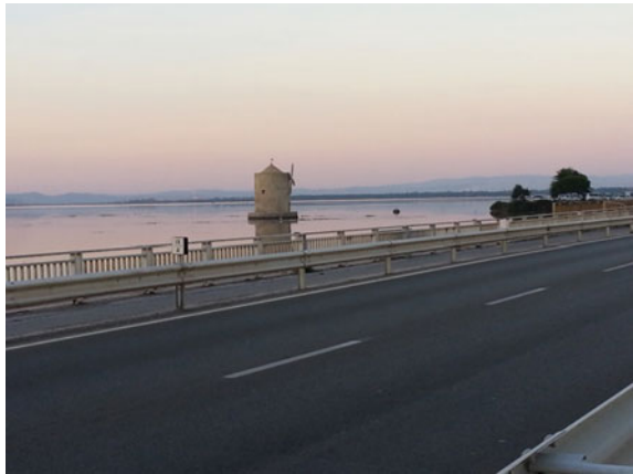
Fig. 5 Photograph of the embankment with the mill in the foreground (Chiavoni 2014)
