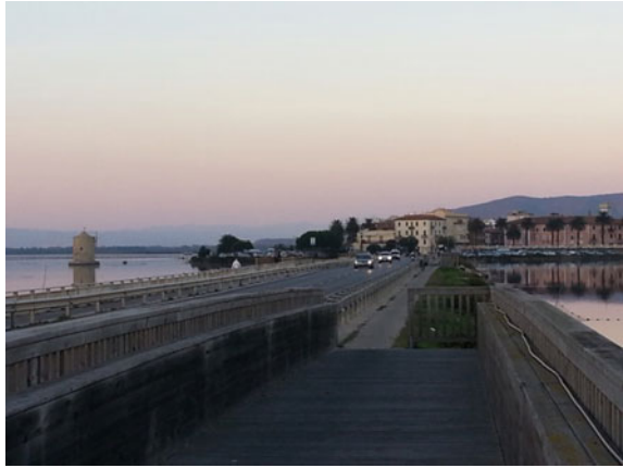
Fig. 4 Photograph of the embankment (Chiavoni 2014)
