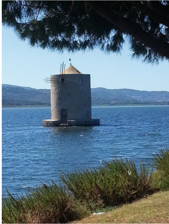
Fig. 11 Photograph of the mill today on the Orbetello Lagoon (Chiavoni 2012)
